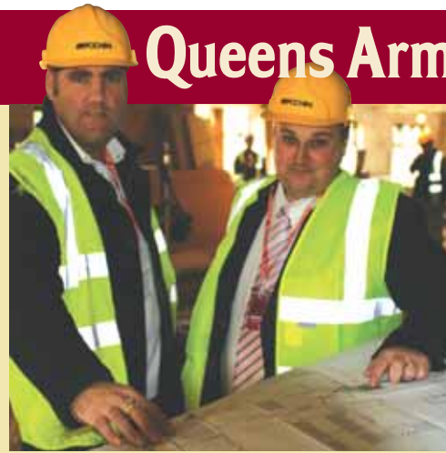
Brian Stokes (L) liaised closely with District Manager Tony Massey throughout the refurbishment
